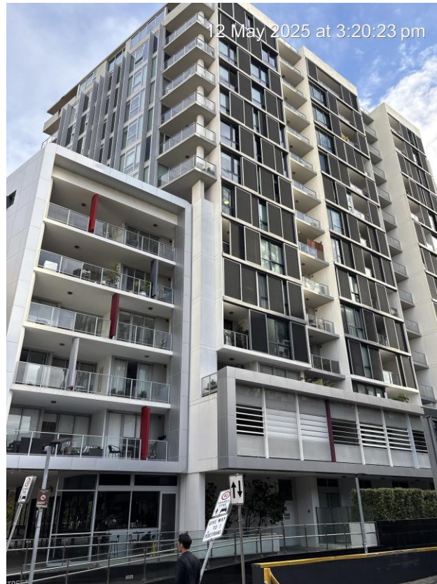
Figure 1: 200-218 Goulburn Street, Surry Hills, viewed from the north-west
